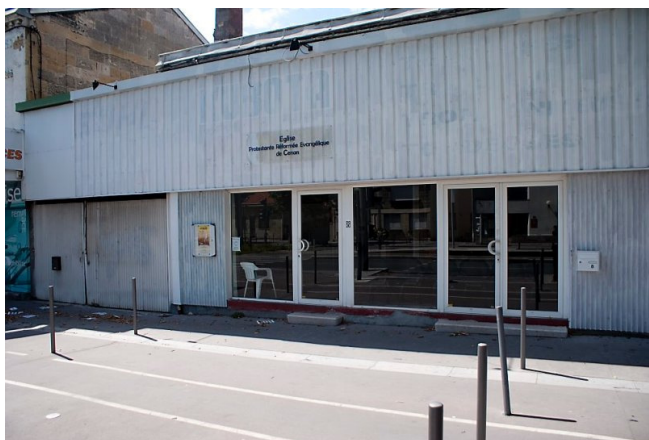
Exterieur van de Eglise Portestante Reformee Evangélique in Cenon (Bordeaux)
